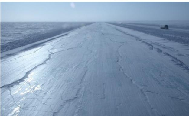
Figure 8. Common longitudinal cracking from wear and tear on the ice road surface
