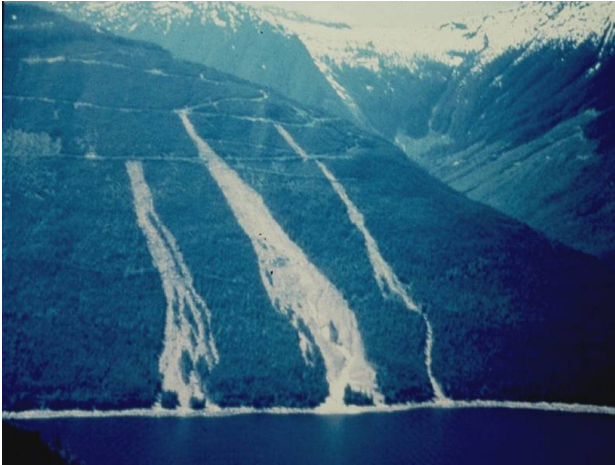
Figure 1. Landslides from roads caused by slope overloading and inadequate drainage.
