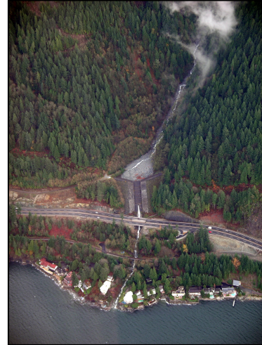
Figure 5. Charles Creek debris basin at work. Notice the debris basin is stopping the debris flow deposit and protecting the Sea to Sky Highway, railway, and homes built on the alluvial fan.
