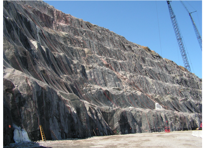
Figure 12. Mesh installation with crane on the slope face
