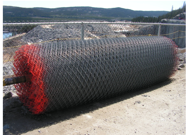
Figure 9 High strength mesh roll to be installed
