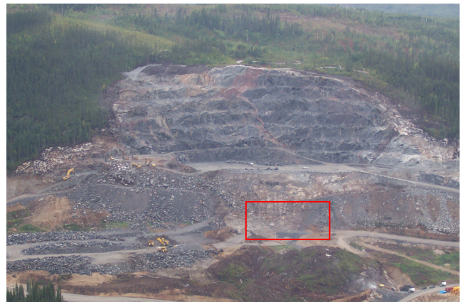
Figure 3. Péribonka spillway excavation. Spillway concrete structure zone in box.
