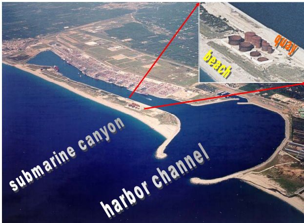
Figure 2. Aerial view of the critical facility.
