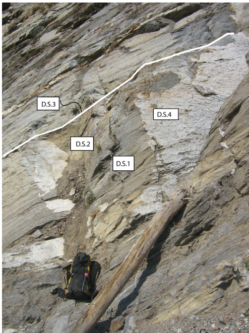
Figure 4: Close-up of the rockmass in the headscarp of the Clanwilliam Landslide highlighting the four major discontinuity sets identified.
