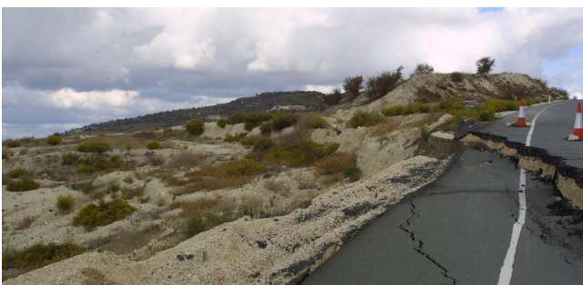
Figure 16. Horseshoe failure.
